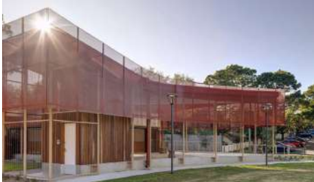
Project: Hurlstone Memorial Reserve Community Centre / Sam Crawford Architects
