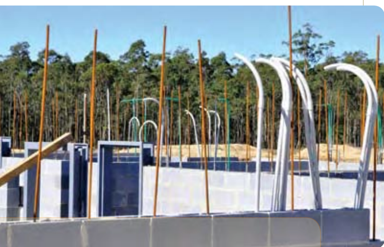
Construction of new correctional centre at Nowra (photo)
