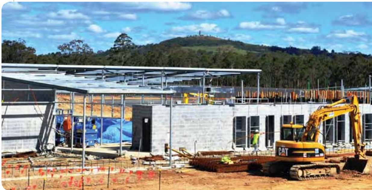
Correctional centre construction site at Nowra
