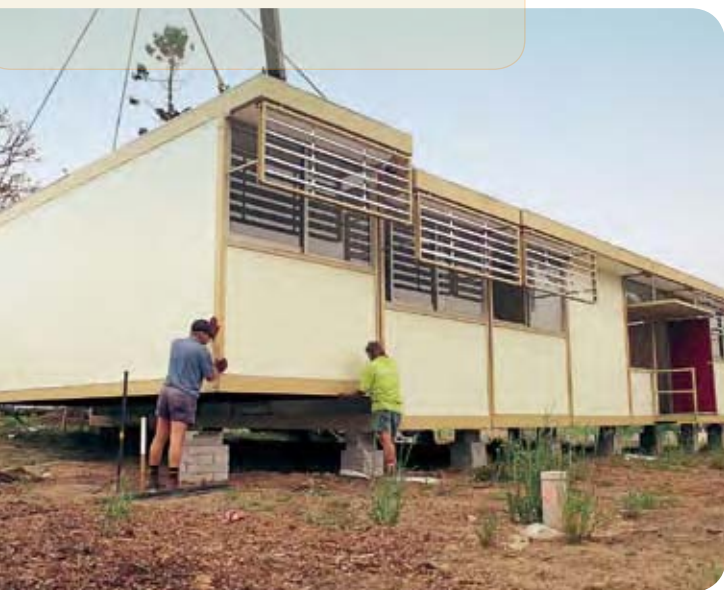
Installation of demountable classroom repaired by inmates at Cessnock Correctional Centre
